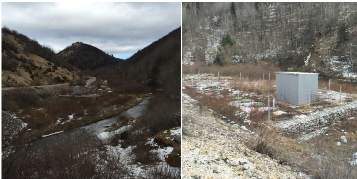
Figure 20. Collector for wastewater treatment along the Rakitnica river (directly in front of its canyon)
