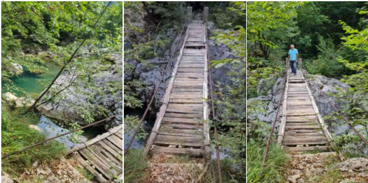
Figure 25. Bridge in the canyon of the Rakitnica river
