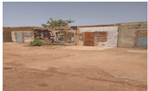
Photo 1. Property affected by the project
